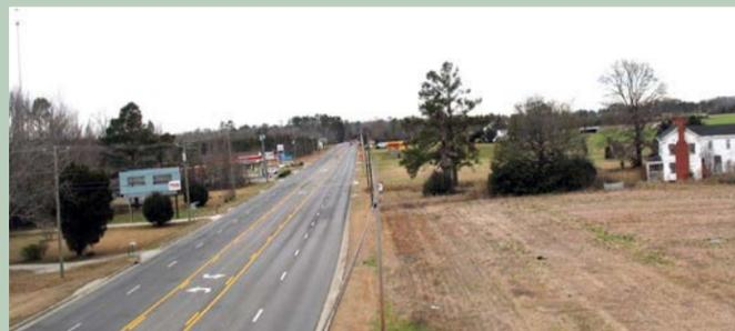
A **median acceleration lane** would aid safe left turns at Waterlily Road and U.S. 158. U-turn bulbs at nearby intersections would also provide additional flexibility for local traffic near the Mid-Currituck Bridge interchange.
